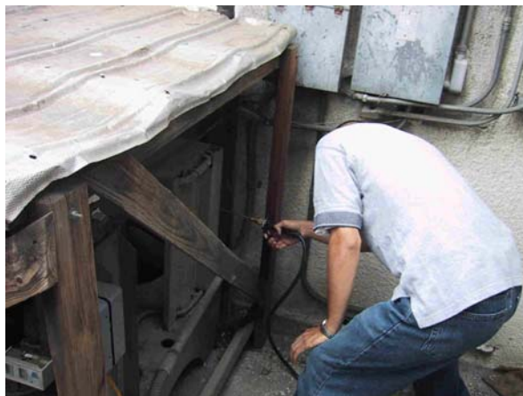
Figure 3. Small Refrigeration System Condenser Coil being cleaned.(This coil has not been cleaned since installation)
