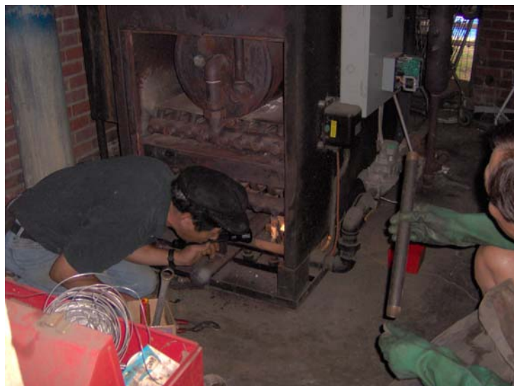
Figure 6. Inspection Before Start of Boiler Tube Cleaning
