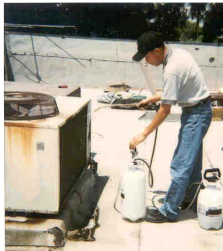
Figure 2. A/C Unit Condenser Coil Being Sprayed Before Cleaning
